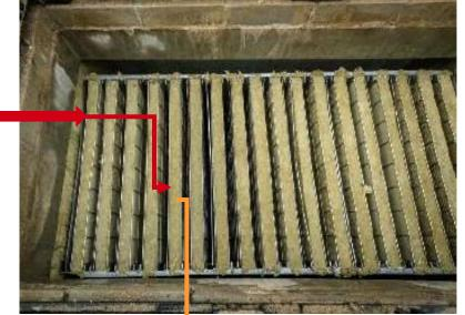
**Lamella filter** Filter > 45µm SS
