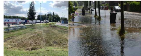
Figure 9.44 Diminished functioning of SUDS. Left: Maintenance with heavy equipment leads to compaction of the soil (Source: https://www.climatescan.org/projects/6915/detail ). Right: insufficient hydraulic capacity of a swale and road flooded with stormwater (source: https://www.climatescan.org/projects/210/detail ).
